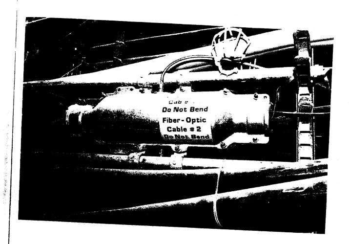
Fiber-optic cable and splice case
